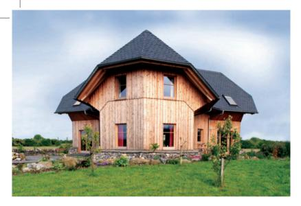
Slate has a layered fabric along which it is readily split, making it ideally suitable as a roofing material. It is capable of being split thinner than other natural roofing materials and therefore has greater coverage per unit weight than other choices. Although there is a large variation in the embodied carbon of natural roofing slates (Table 1) its embodied carbon value is at most 16% of that of other roofing materials.
